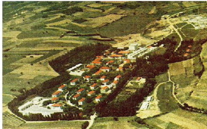
VINČA Institute – aerial photo
