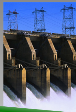
Hydroelectric Power Station
